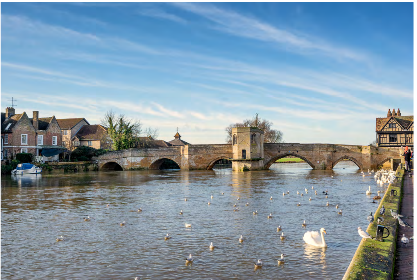
Figure 6: St. Ives Bridge over the River Great Ouse 11
